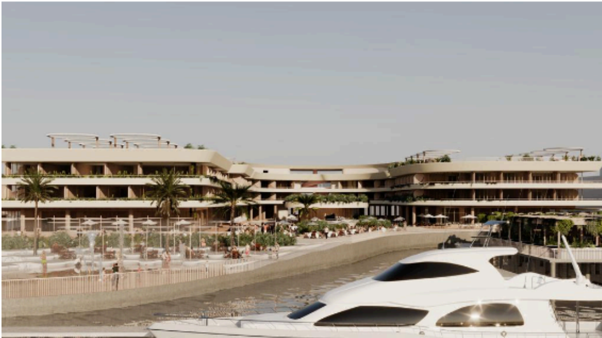
A render of the Ritz Carlton, Gold Coast, which is slated to open in 2026. Picture: Supplied
